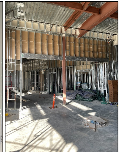
Café Entry Framing – 1 st Floor
