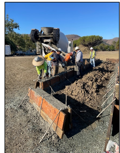
Site Electrical Trench & Concrete Curbs at Parking Lot 4
