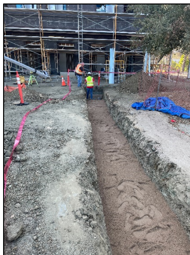
Site Electrical Trench & Concrete Curbs at Parking Lot 4
