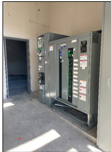
Electrical Switchgear
