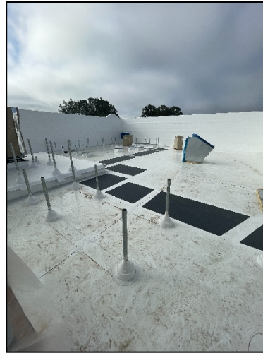
Roof Walk Pad Installation
