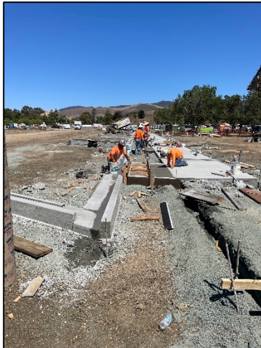
Parking Lot 4 Curbs, Pedestrian Flatwork, Demo, & Earthwork
