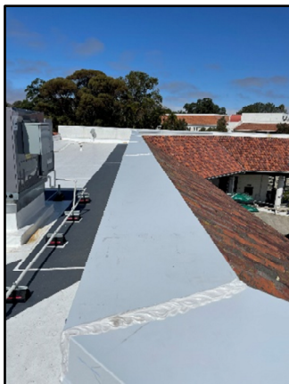
New Parapet Cap
