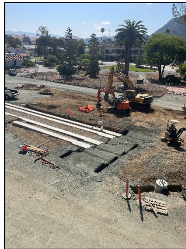
Terraced Seating Stair Footings Parking Lot 4 Curb Forms
