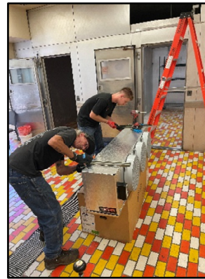
Refrigerator Evaporators
