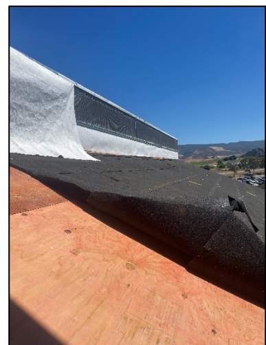
Mansard Roof Parapet Wall Exterior Lath
