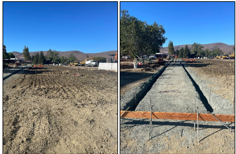
Parking Lot 4 Demo & Pedestrian Flatwork
