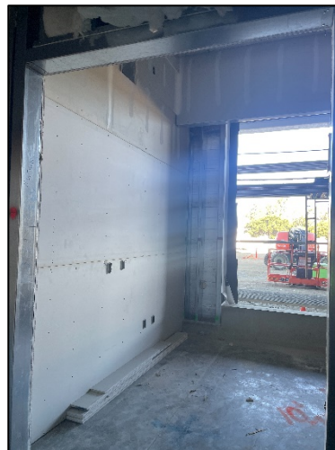
1 st Floor Interior Insulation & Drywall
