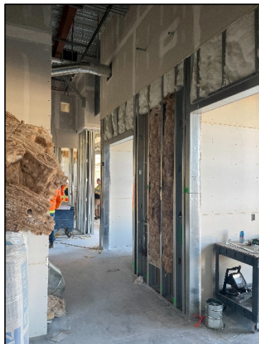
1 st Floor Interior Insulation & Drywall
