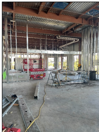
2 nd Floor Interior Framing Board Room Entry
