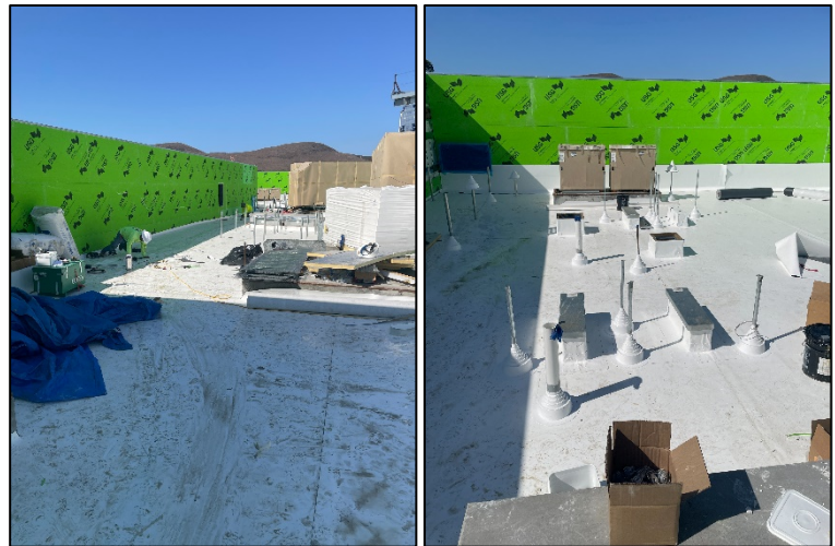
Single Ply Roofing Installation
