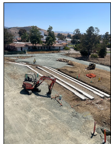
Exterior Hardscape Footings
