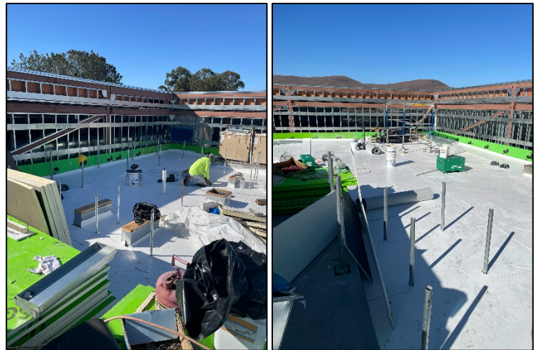
Single Ply Roofing Installation
