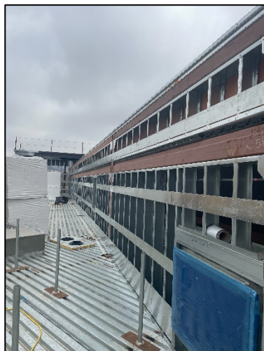
Roof Parapet Wall Framing
