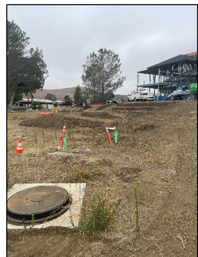
Exterior Hardscape Footings
