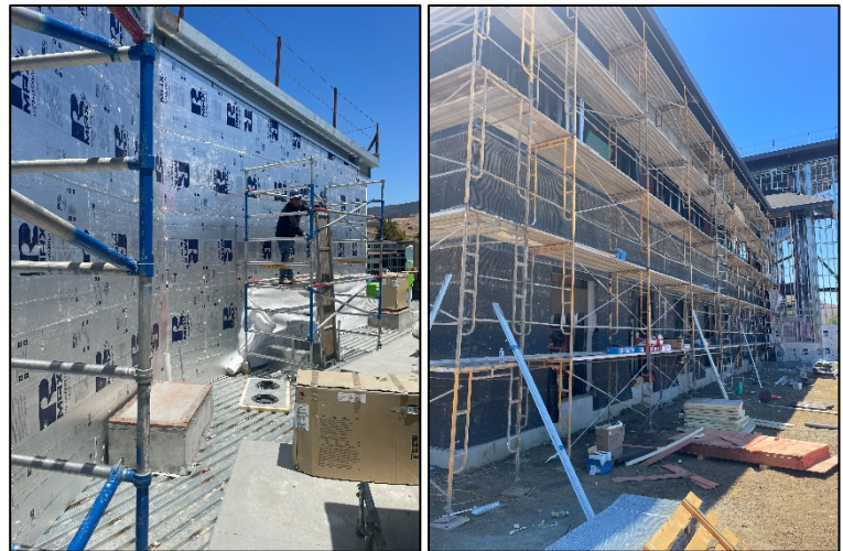
Exterior Rigid Insulation & Lath
