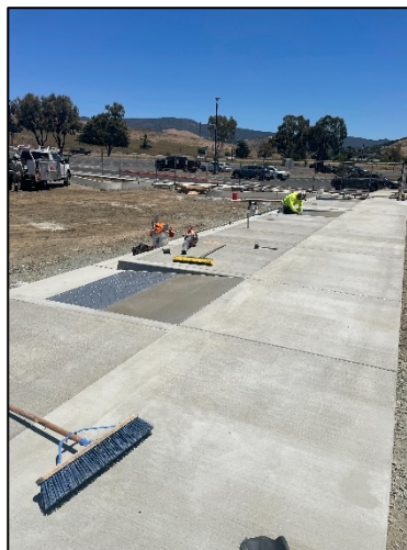
Parking Lot 3 Flatwork
