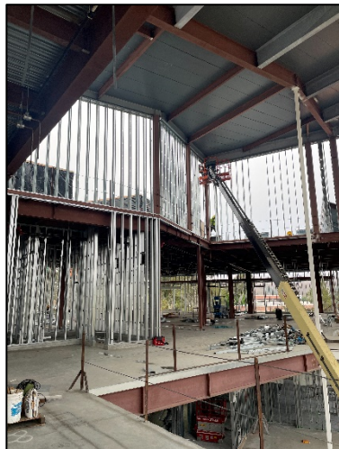
High Roof Wall Framing
