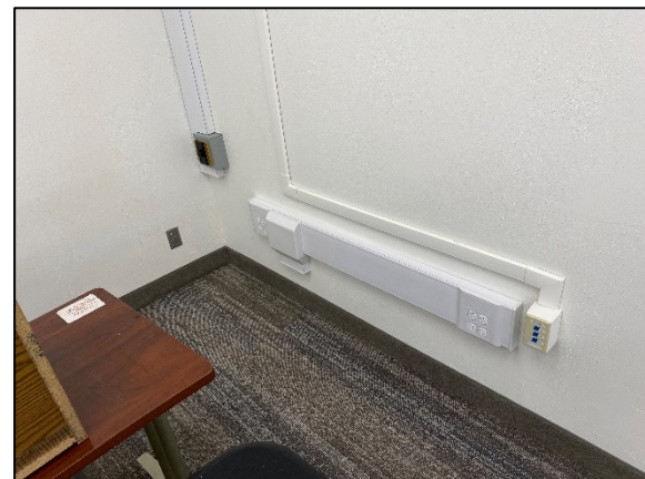
4100: Wire Molding Completed
