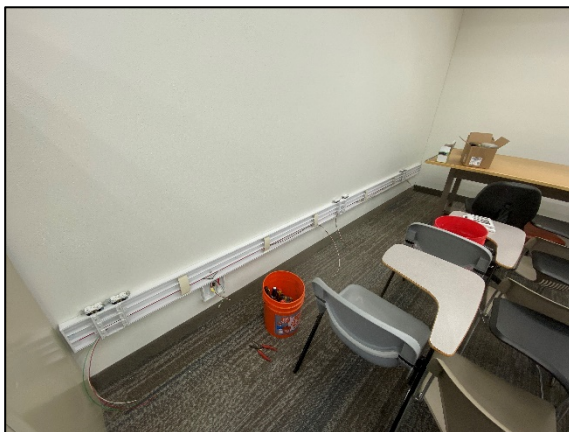
4100: Wire Molding In Progress
