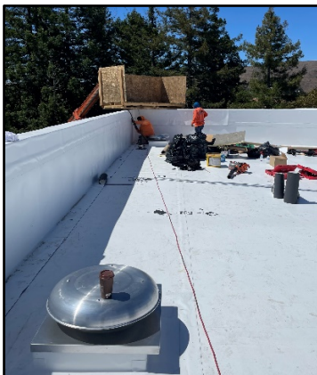
New Single Ply Parapet 5200
