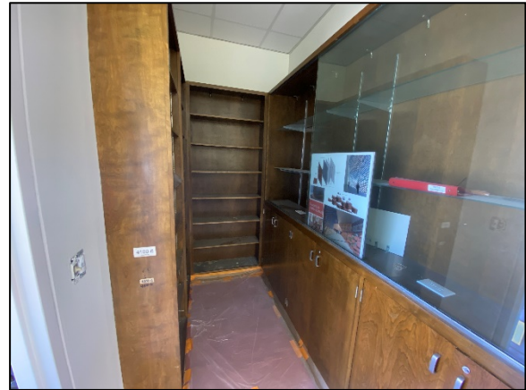
4100: Existing Cabinets Refinished
