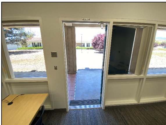
4100: Door Frames Painted
