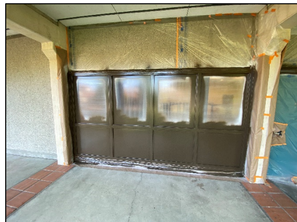
Paint at Exterior Storefront
