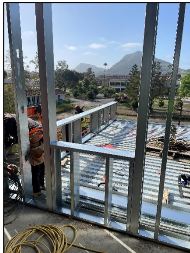
[ 2 nd Floor Exterior Framing ]
