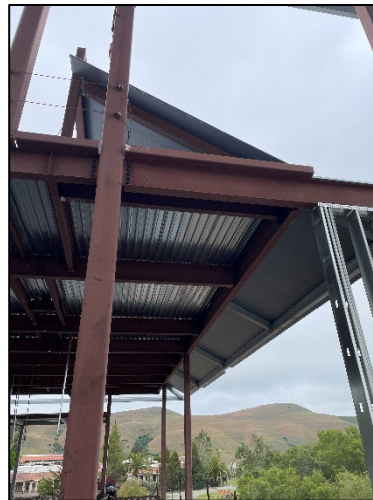
[ Mansard Roof Metal Deck ]
