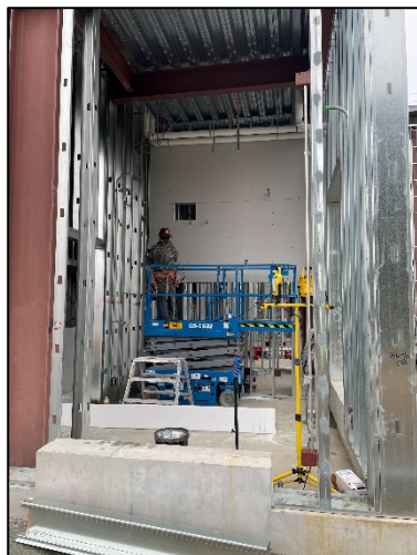
[ 1 st Floor Int. Drywall ]
