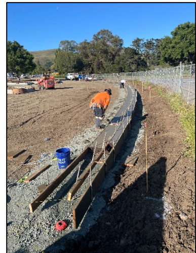
[ Parking Lot 4 Curb ]
