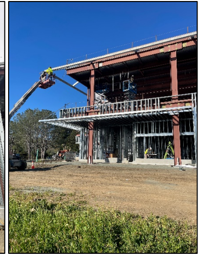
[ Mansard Roof – Steel ]
