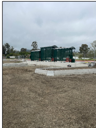
[ Bus Shelter Installation ]
