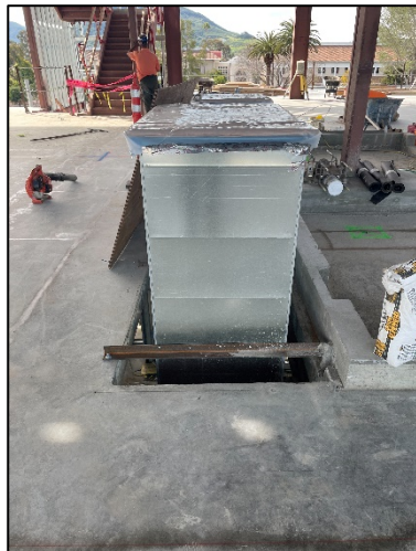
[ HVAC Duct Rough-In ]
