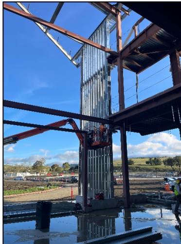
[ Metal Wall Stud Installation ]
