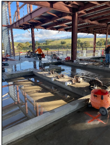
[ 2 nd Floor Concrete Wall Curbs ]
