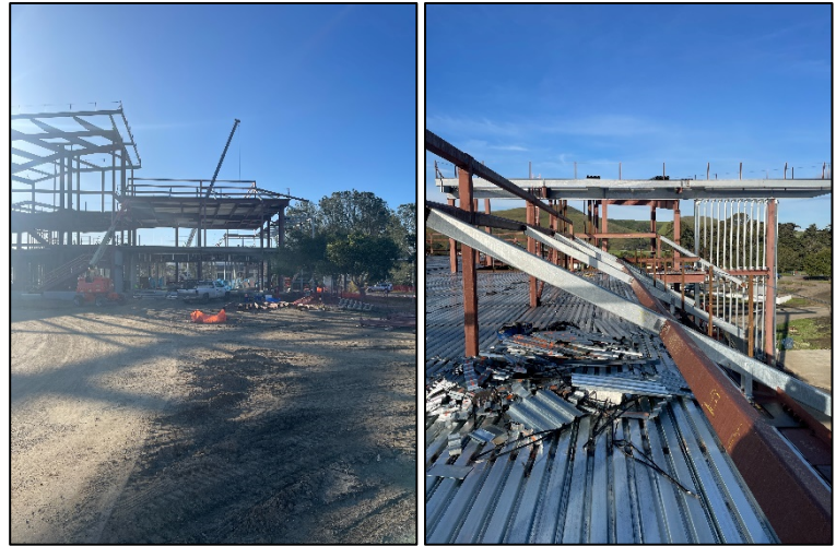
[ Mansurd Roof – Structural Steel ]
