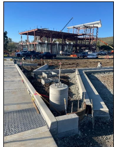
[ Parking Lot 3 Curb & Gutter ]
