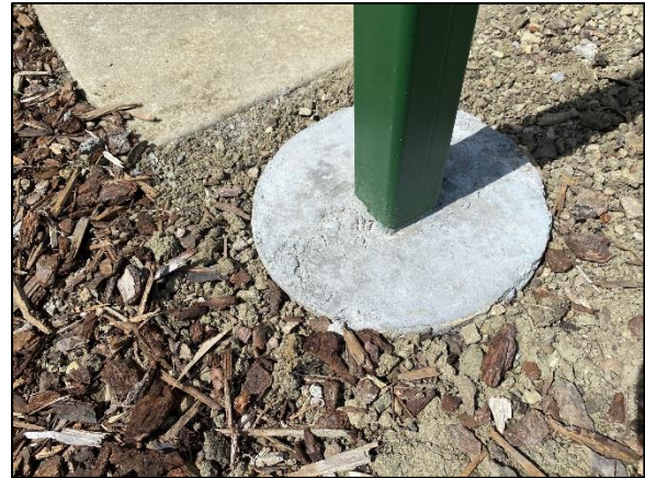
Footing Prior To Sack & Patch
