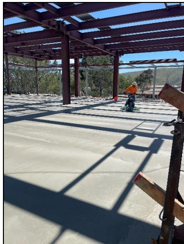
[ 2 nd Floor Concrete Deck ]
