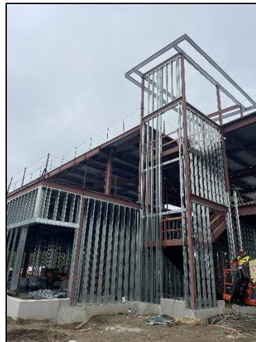
[ Metal Wall Stud Installation ]
