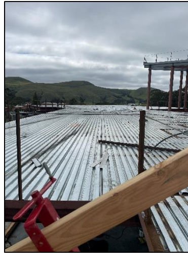
[ Metal Deck Installation – Roof Level ]
