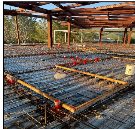
2 nd Floor Deck Sleeves
