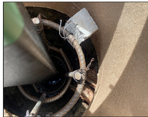
Sign Footing w/ Rebar Cages
