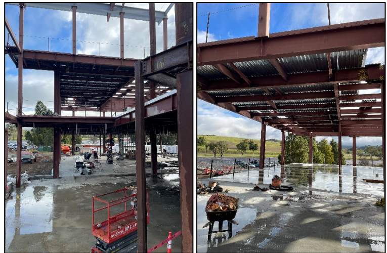
[ Metal Deck Installation – Roof Level ]
