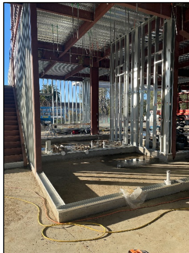
[ Metal Wall Stud Installation ]
