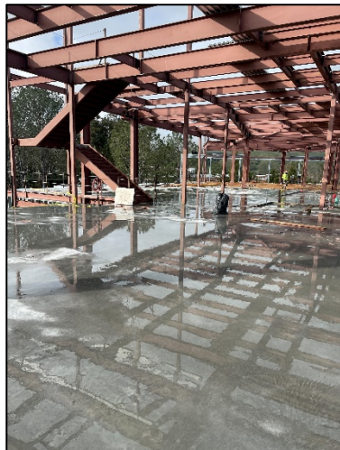
[ 2 nd Floor Concrete Deck ]
