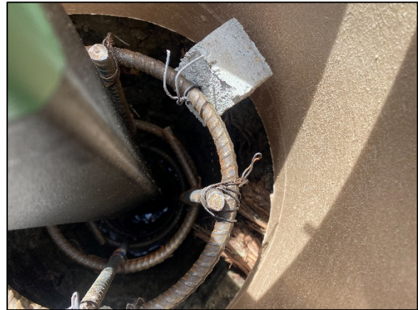
Footing Rebar Cages
