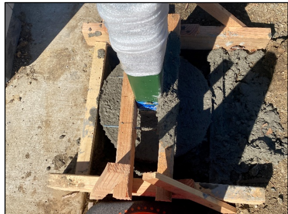
Footing Prior to Finish Work
