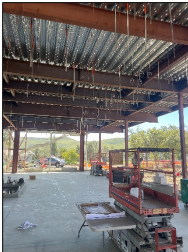
[ HVAC & Fire Sprinkler Support Hangers ]
