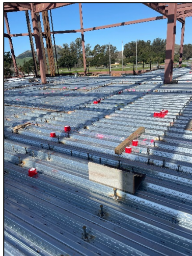
[ 2 nd Floor Deck Penetration Boxes ]
