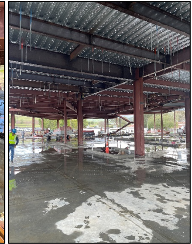
[ HVAC Duct Support Strap Installation ]
