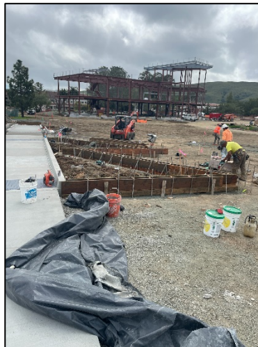
[ Parking Lot 3 Curb Installation & Pedestrian Flatwork ]
