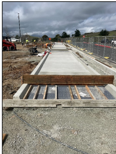
[ Parking Lot 3 Curb Installation & Pedestrian Flatwork ]
