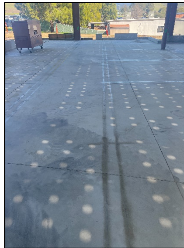
[ Wall Layout For 2 nd Floor Deck Utility Install ]
