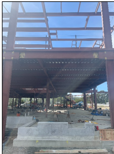
[ 2 nd Floor Metal Deck Installation ]
