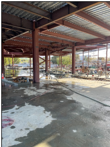
[ 2 nd Floor Metal Deck Installation ]
