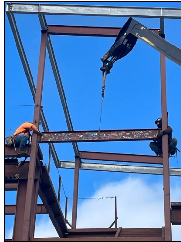
[ Signed Beam Install ]
