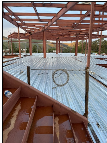
[ 2 nd Floor Metal Deck Installation ]
