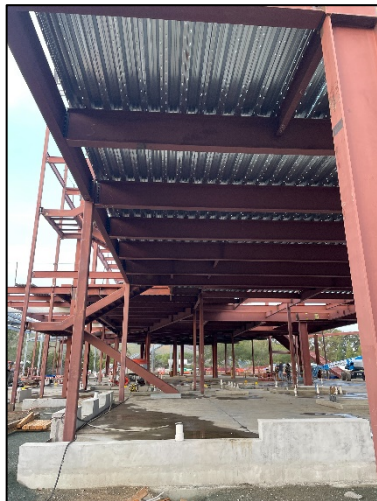
[ 2 nd Floor Metal Deck Installation ]
