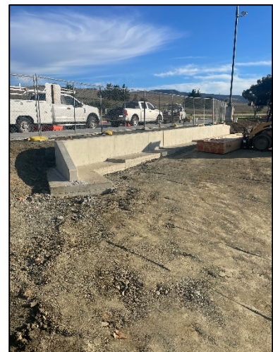
[ Parking Lot 3 Expansion – Retaining Wall ]
