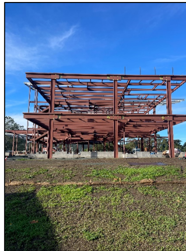
[ Structural Steel Erection ]
