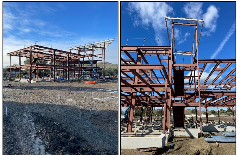
[ Structural Steel Erection ]
