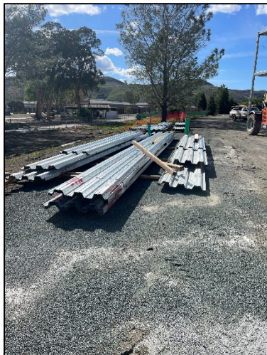
[ Metal Deck Staging ]
