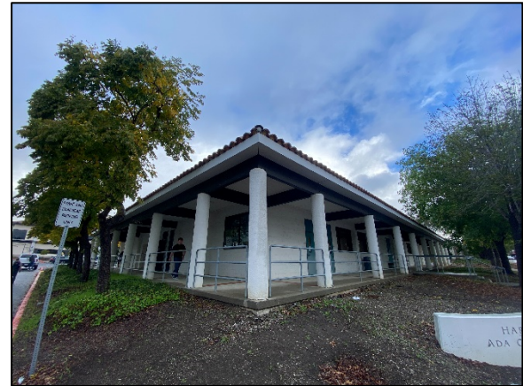
Demo & Patch Bldg. 2500
