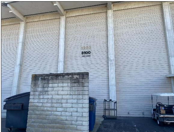
Demo & New Install - 3100
