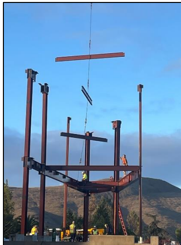
Iron Workers Setting Steel
