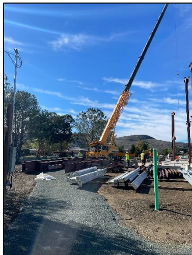
Steel Material Staging
