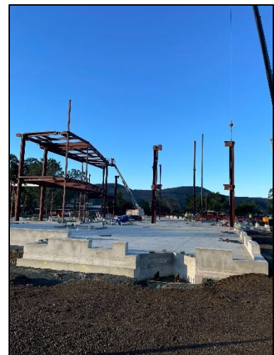
Iron Workers Setting Steel
