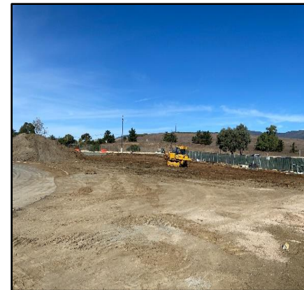
Parking Lot 3 Grading
