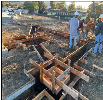
Pad Footings & Tie Beams
