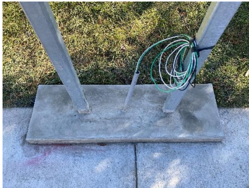
Footings Prior to Sacking
