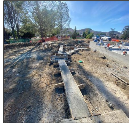
Pad Footings & Tie Beams
