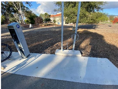
Footing after Sacking
