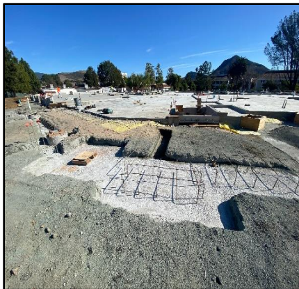
Perimeter Wall Curb
