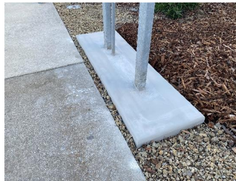
Footings after Sacking
