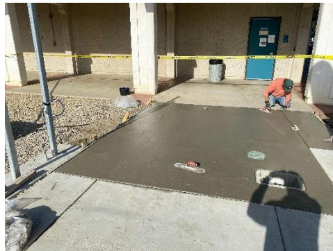
Flatwork at Location E-06
