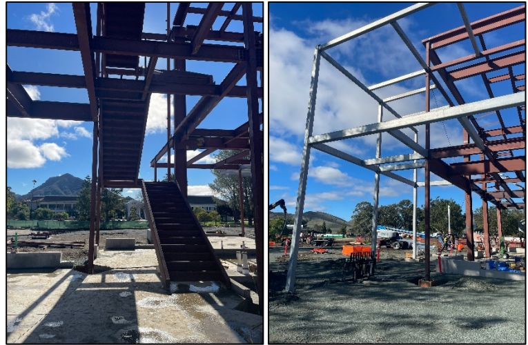
[ Structural Steel Erection ]
