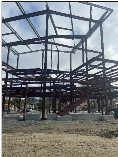
[ 1 st Floor Lobby Stairs ]
