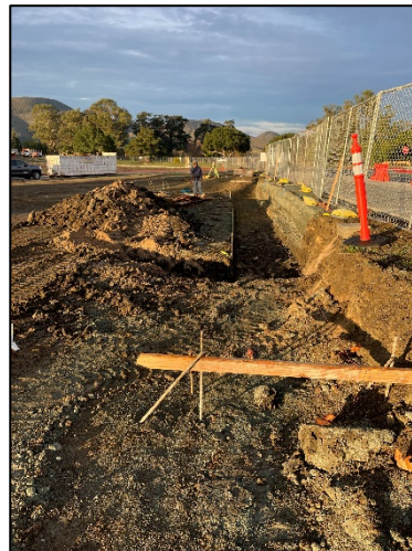
[ Parking Lot 3 Expansion – Retaining Wall ]
