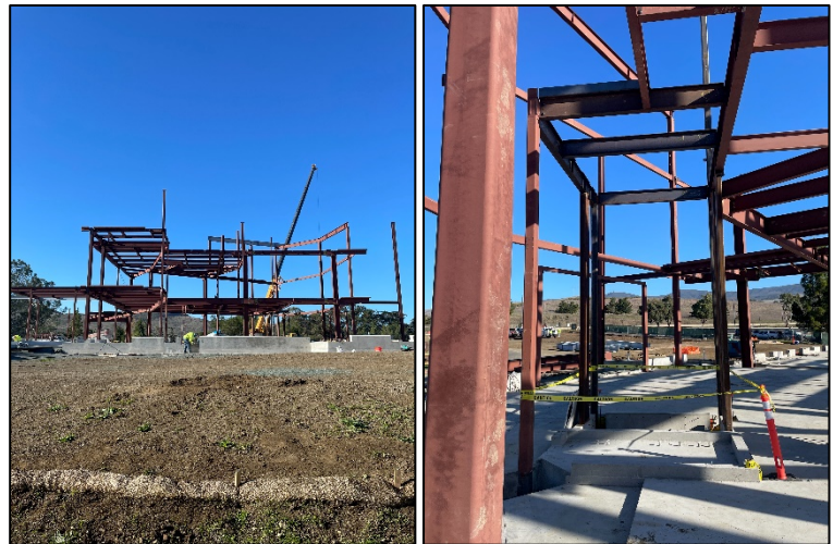
[ Structural Steel Erection ]
