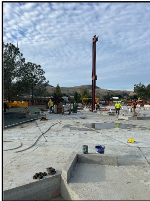
[ 1 st Structural Steel Column Set ]
