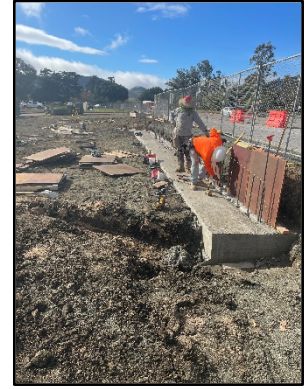
[ Site Retaining Wall – Lot 3 ]
