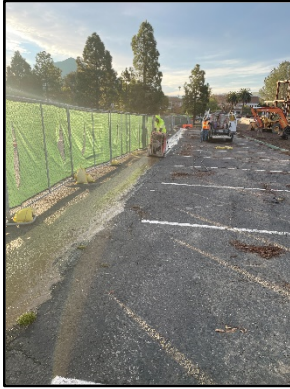
[ Asphalt Saw-Cut Lot 3 Expansion ]
