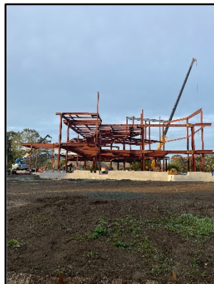
[ Structural Steel – Erection Activity ]
