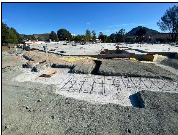
Under-Slab Footings
