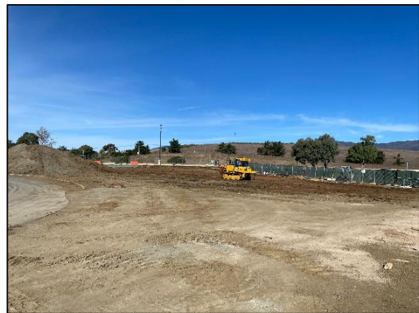
Parking Lot 3 Grading
