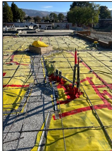
Under Slab Vapor Barrier & Rebar (West Side)
