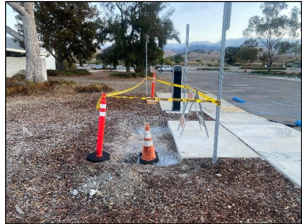
Concrete Demo E-01
