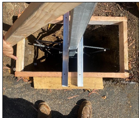
Formwork and Rebar
