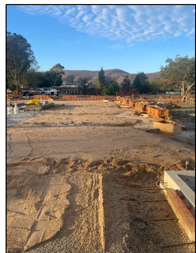
Under Slab Sand (West Side)
