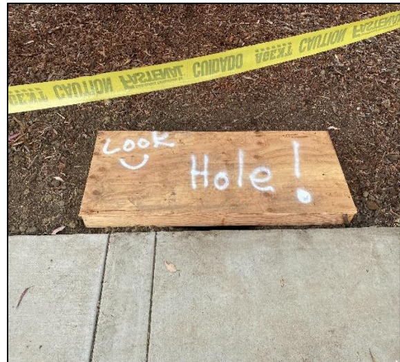
Directory Sign Footing Location
