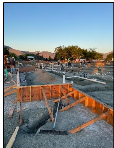
West Perimeter Form Boards
