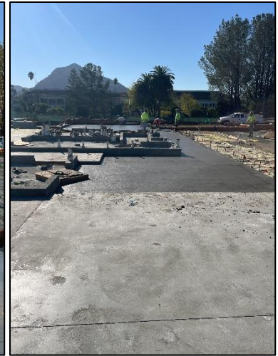
Slab On Grade (East Side)
