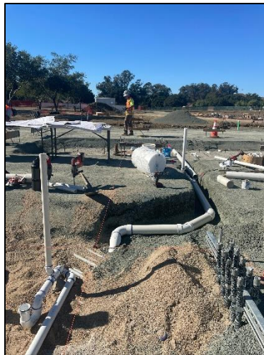
Under Slab Plumbing (West)
