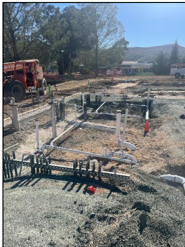
Under Slab Plumbing (West)
