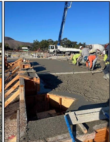
Slab On Grade (East Side)
