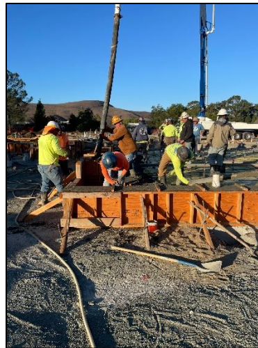
Perimeter Wall Curb (East Side)
