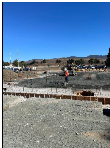
Underslab Base (West Side)
