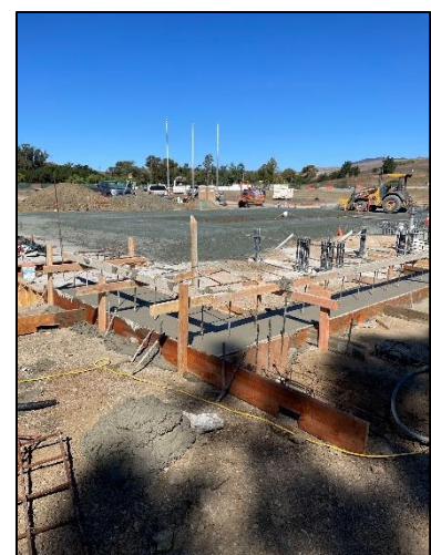
West Perimeter Ftg. Concrete
