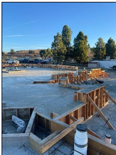
Slab On Grade (East Side)
