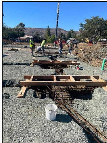
Pad & Tie-Beam Concrete
