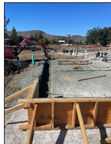
West Perimeter Footing
