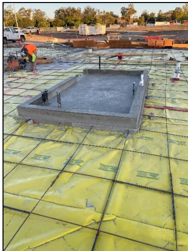
Elect. Room Curb & SOG
