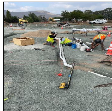
Under-slab Plumbing
