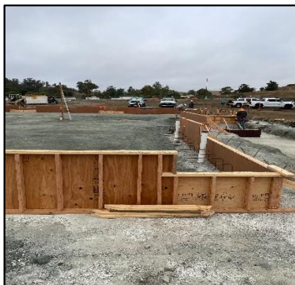
Perimeter Concrete Formwork
