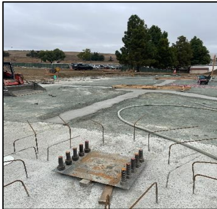
Pad & Tie Beam Concrete
