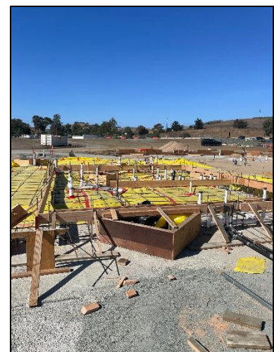
Under Slab Vapor Barrier
