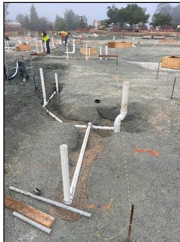
Under Slab Plumbing
