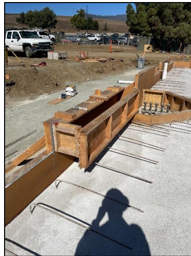
Bldg. Perimeter Wall Forms
