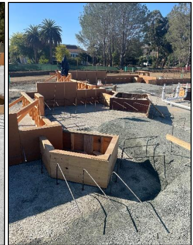
Bldg. Perimeter Wall Forms
