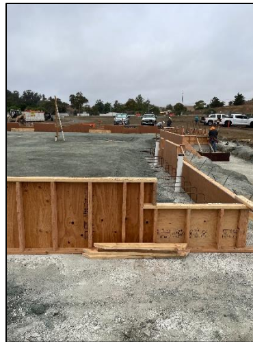
Bldg. Perimeter Wall Forms
