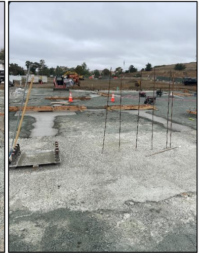
Pad Footing & Tie Beam
