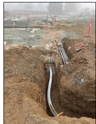
Site Electrical into Bldg.
