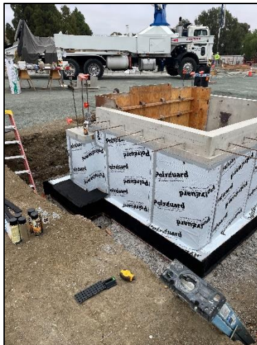
Elevator Pit Waterproofing
