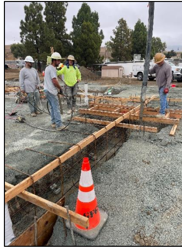
Pad Footing & Tie-Beam
